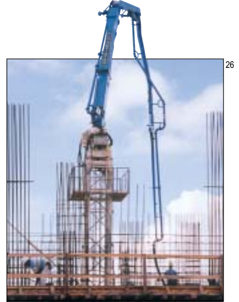
Inside Climbing via Crane or Hydraulics
